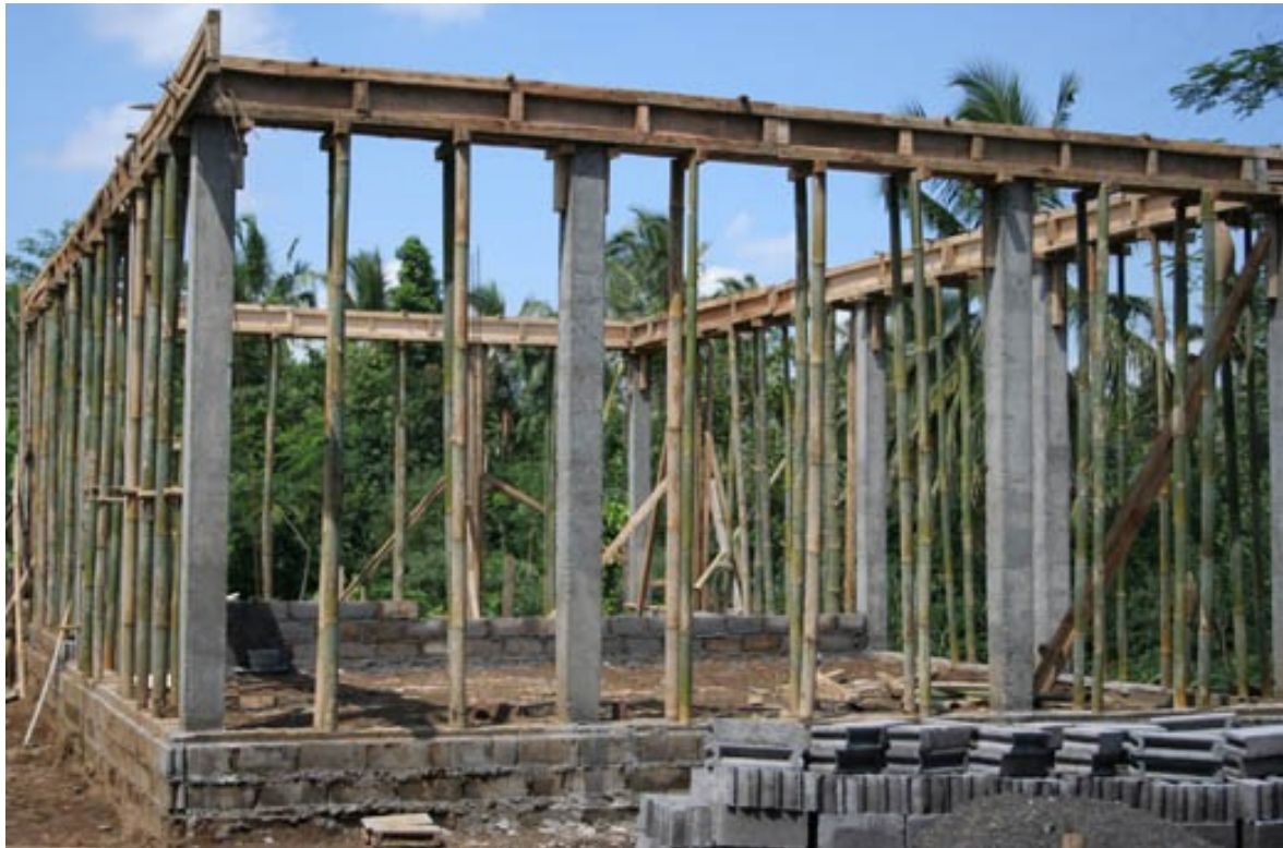
(Tourist place under construction)
